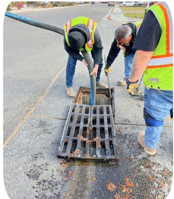
Streets crew cleaned all storm drain catch basins to remove sediment and prevent blockages.
