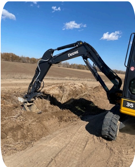
Streets crew cut a swale to help with water erosion and cleaned out the irrigation ditch on the Befus property.
