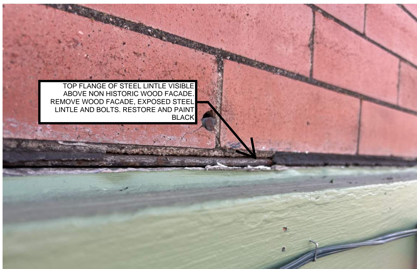
FRONT FACADE STEEL LINTLE PHOTOS NOT TO SCALE
